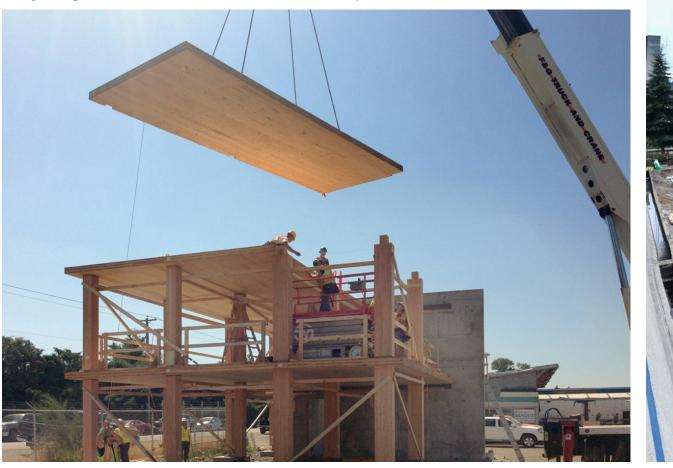
July 2015 erection of mass wood structural mockup
